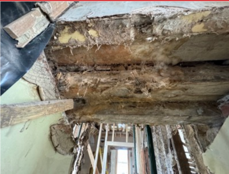
LINTELS TO MASONRY WALL
