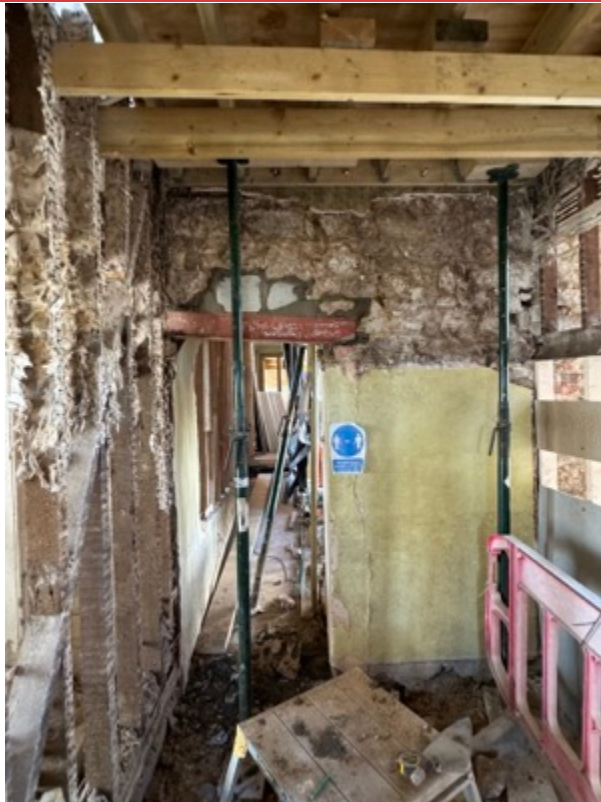
TEMPORARY STEEL INSTALLED TO REPLACE ROTTEN TIMBER LINTEL
