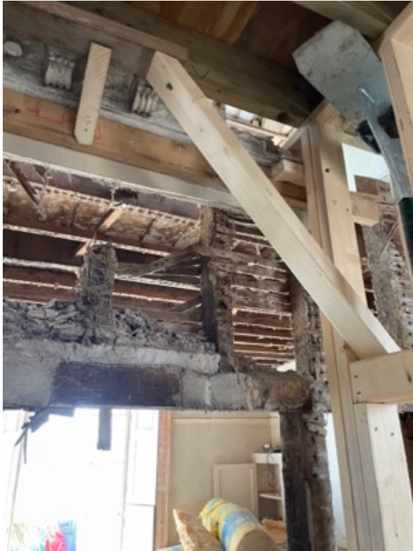
SUPPORTS INSTALLED TO STABILISE WHILST WALL FRAMING REMOVED
