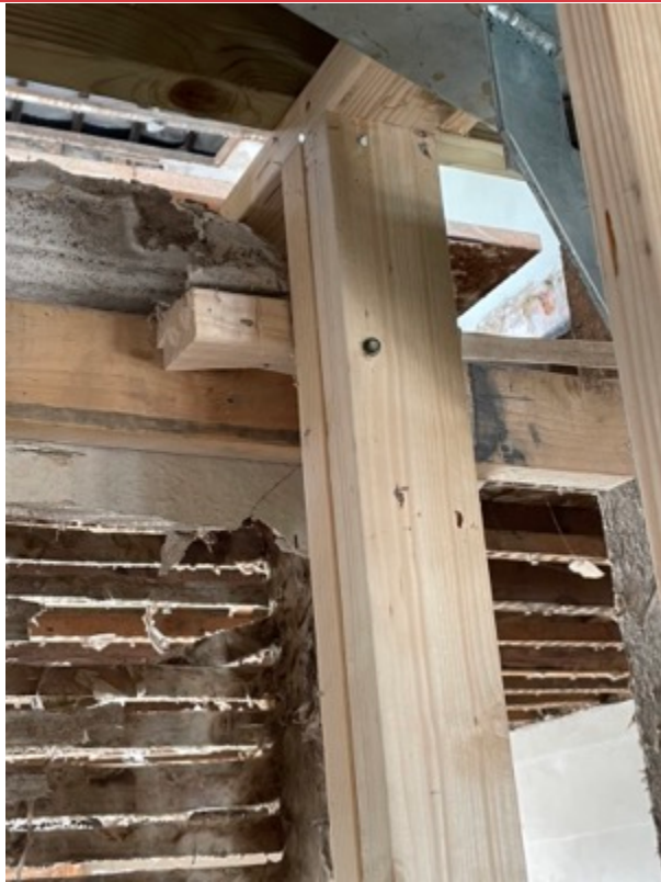
AS ABOVE SUPPORT FIXED TO NEW WALL INSTALLATION
