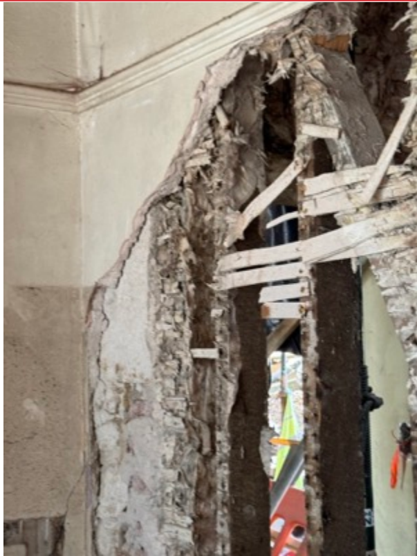
FLAT 2 LOOKING TOWARDS MASONRY WALL
